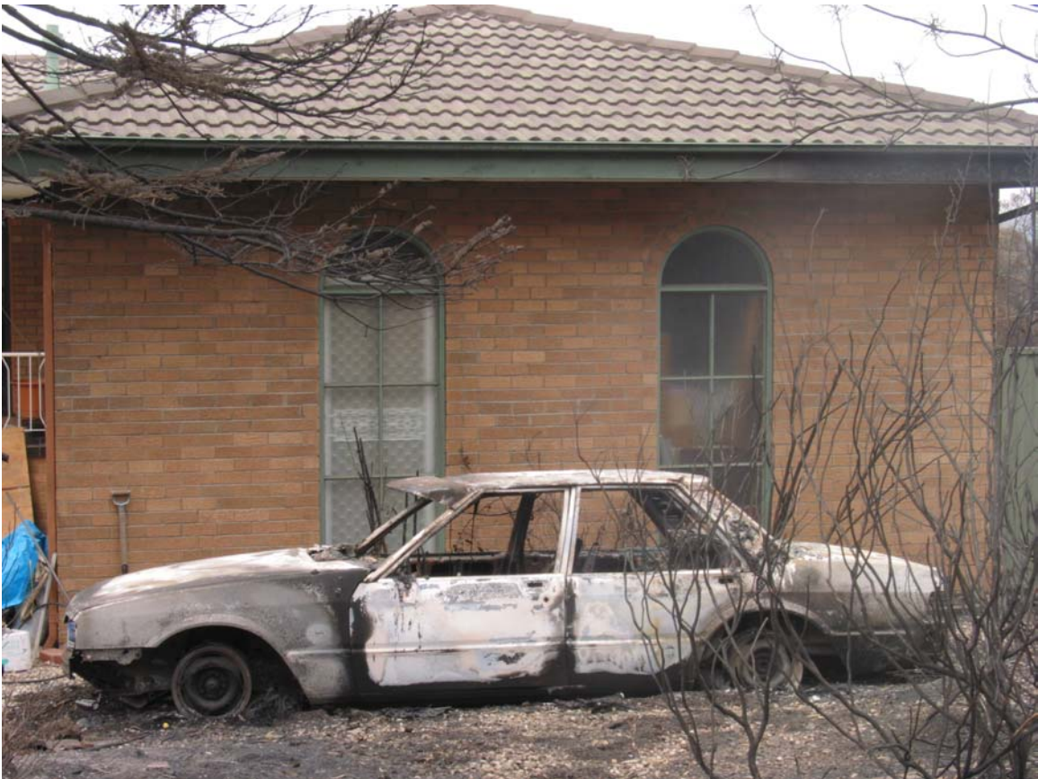
Figure 11. Other example of radiant heat impact due to vegetation and car fire (86 Somerset St)
