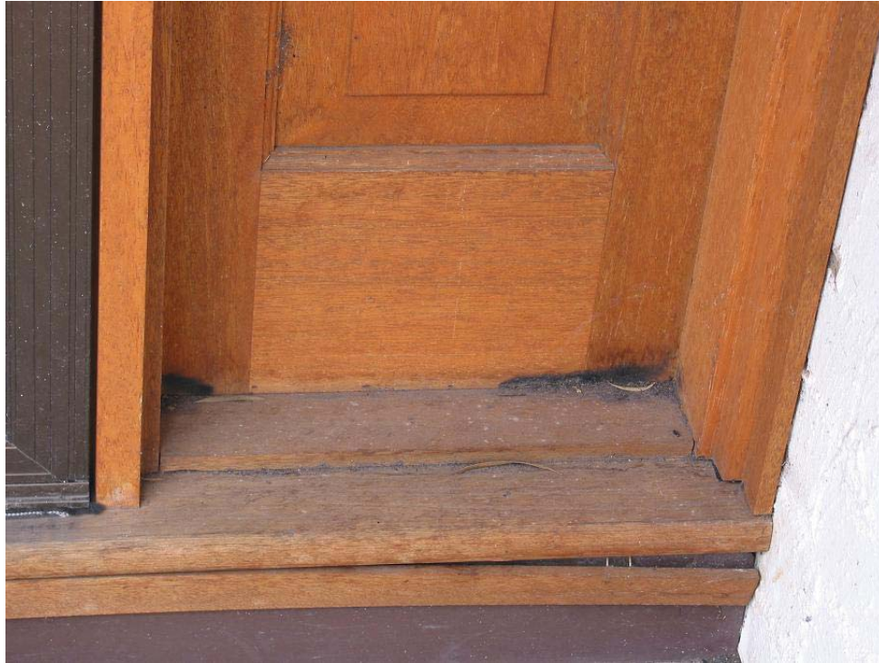
Figure 23. Ember attack on a door (re-entrant corner)
