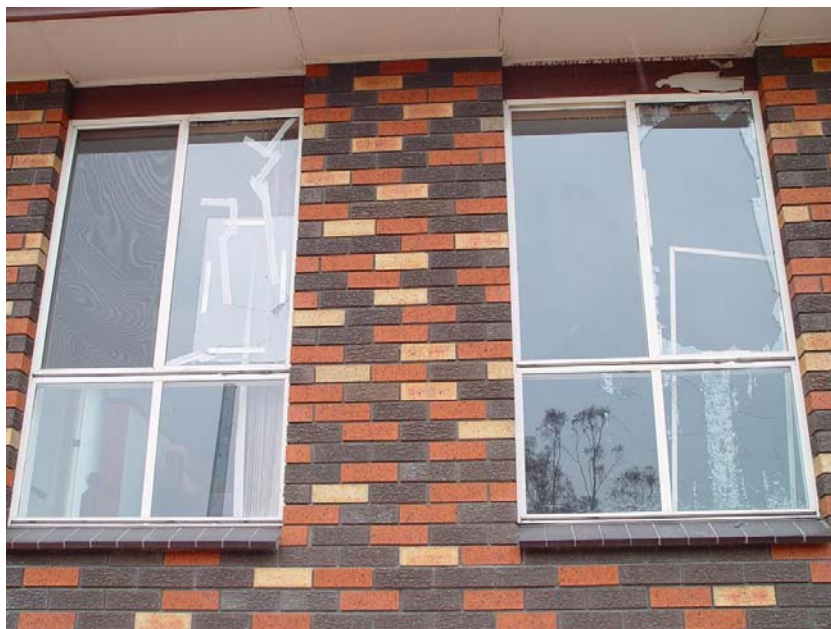
Figure 9. Broken and cracked windows from radiant heat from neighbouring house and fences (73 Somerset St)
