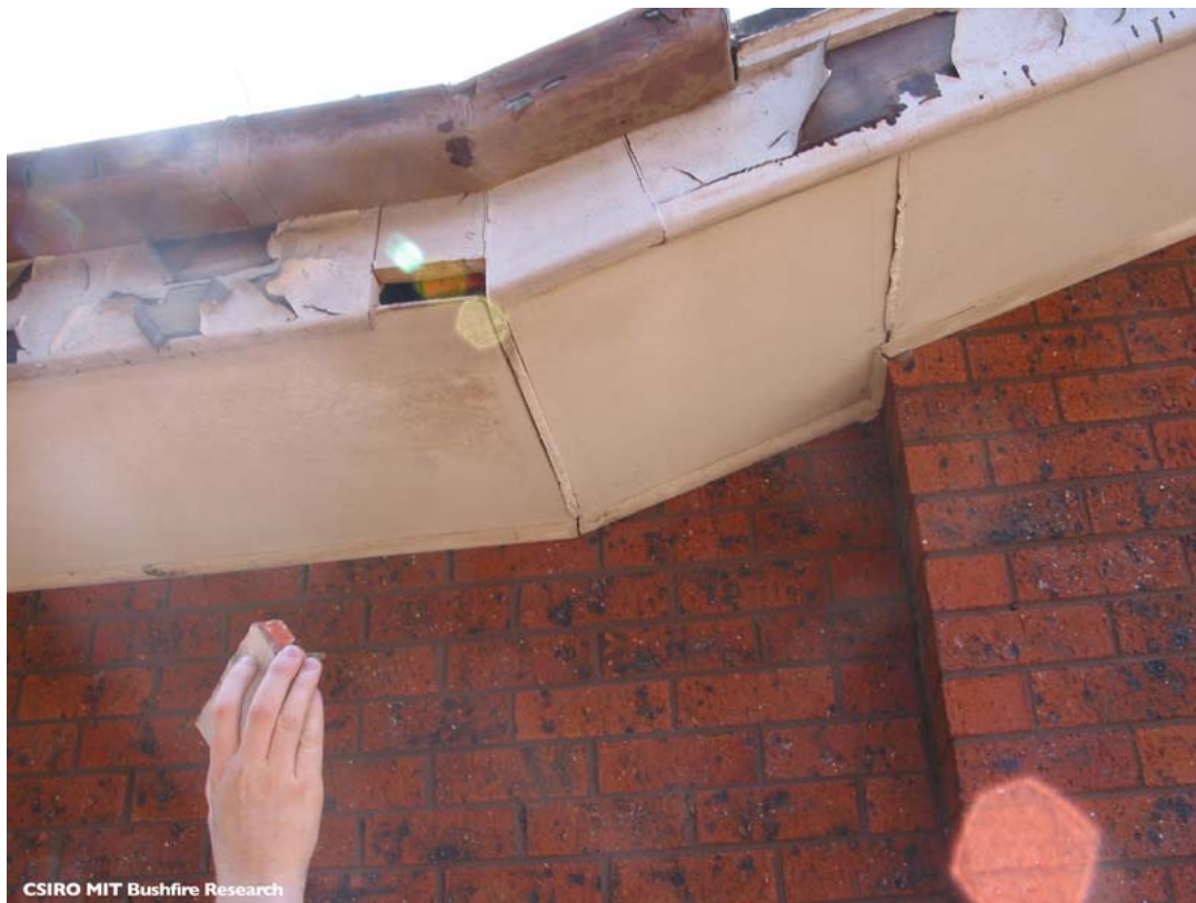
Figure 36. Eaves damage due to radiant heat from adjacent fence and vegetation
