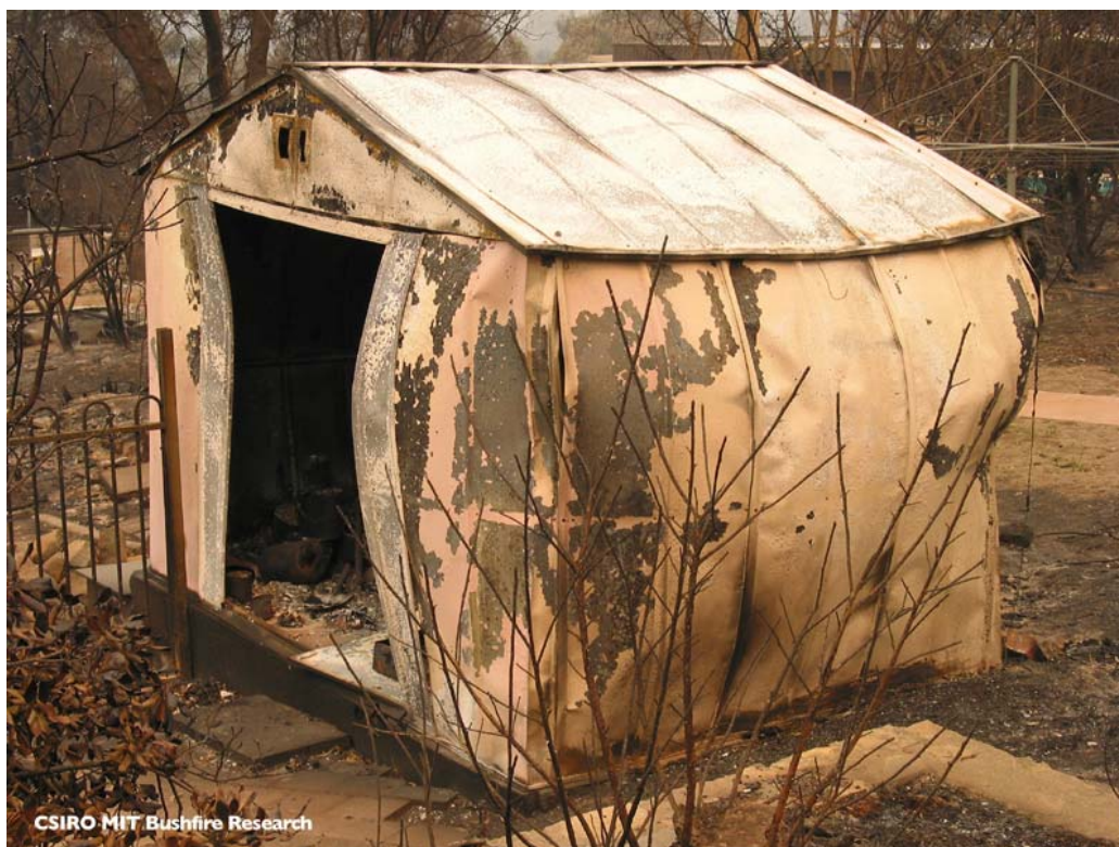
Figure 41. Shed fire damage
