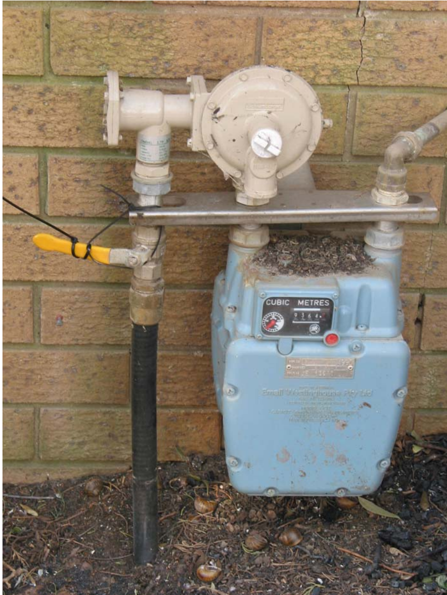
Figure 48. Flexible gas line supply to gas meter
