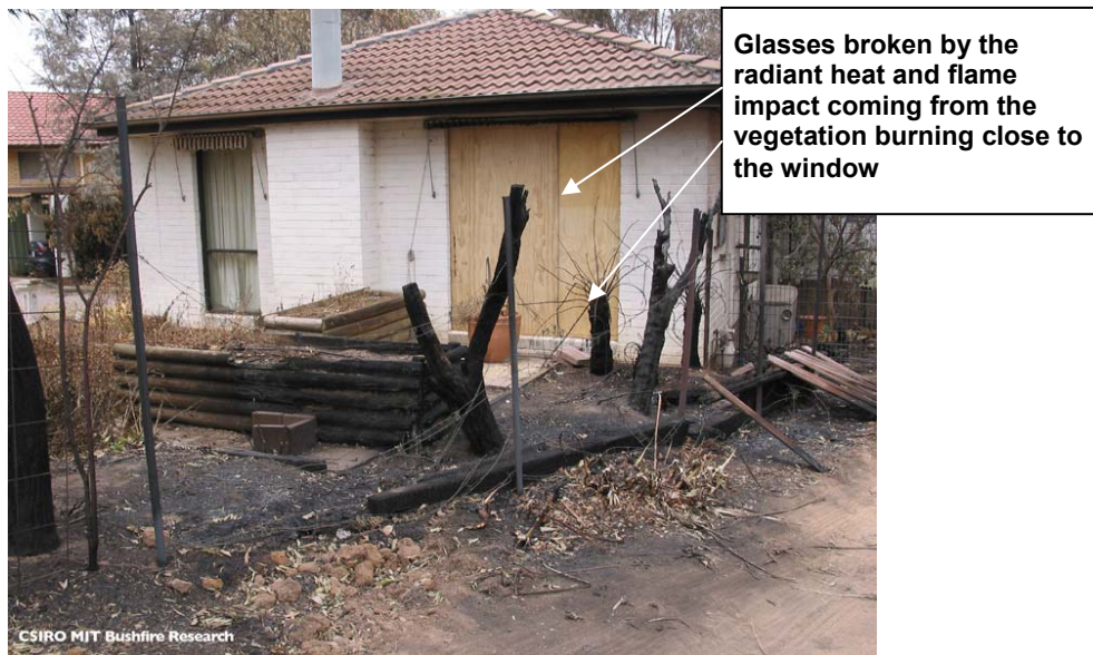
Figure 45. Local fuel impact on a structure
