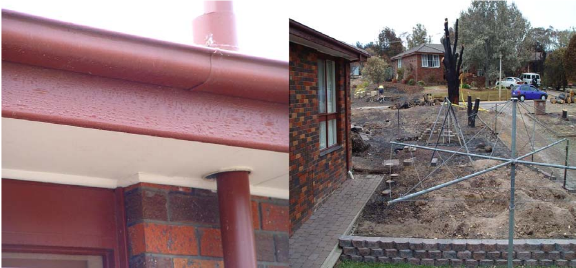
Figure 10. Radiant heat impacts on eaves from surrounding vegetation (73 Somerset St)
