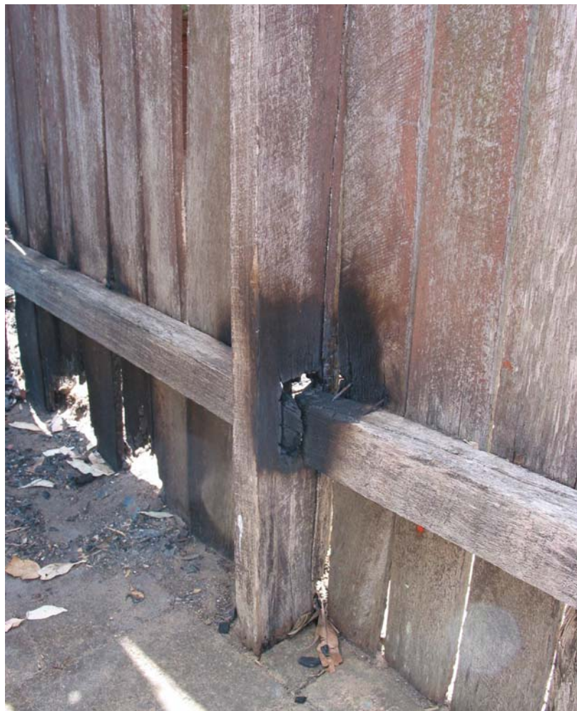
Figure 46. Ember attack on fence (with intervention)
