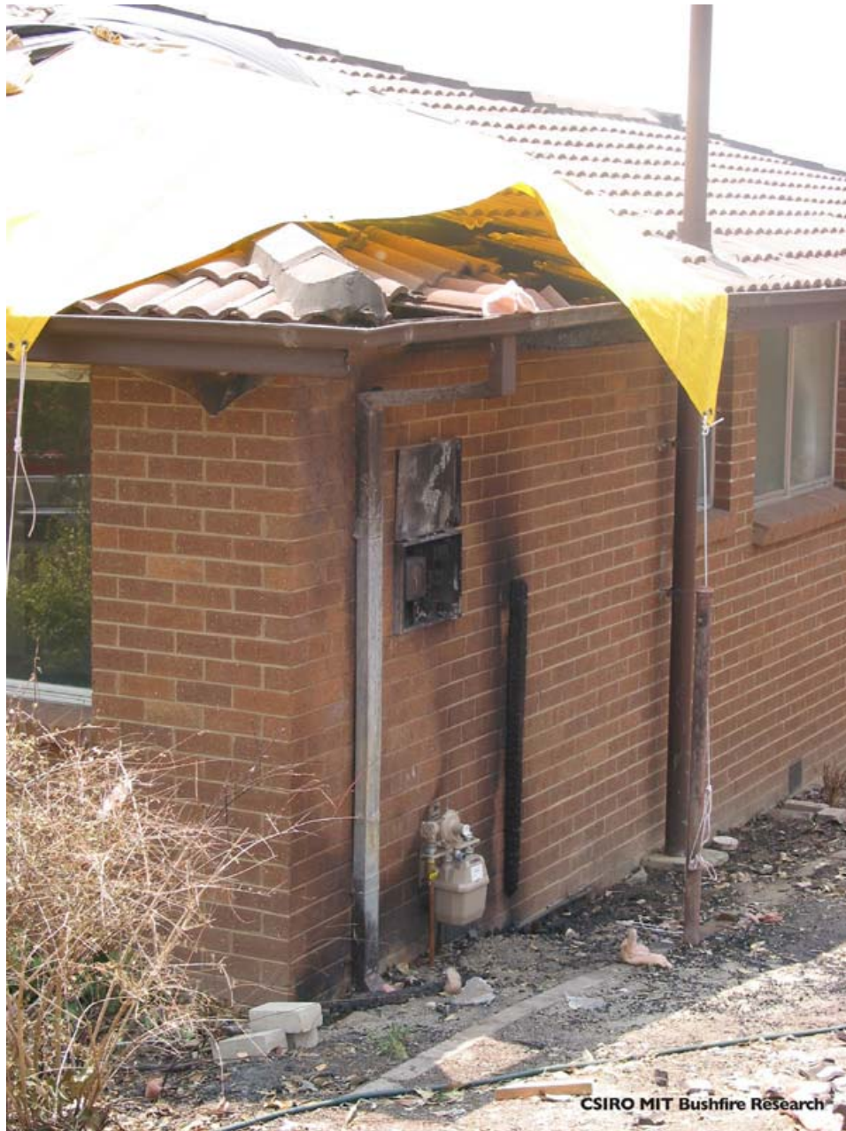
Figure 49. Gas meter flaring attack on eaves
