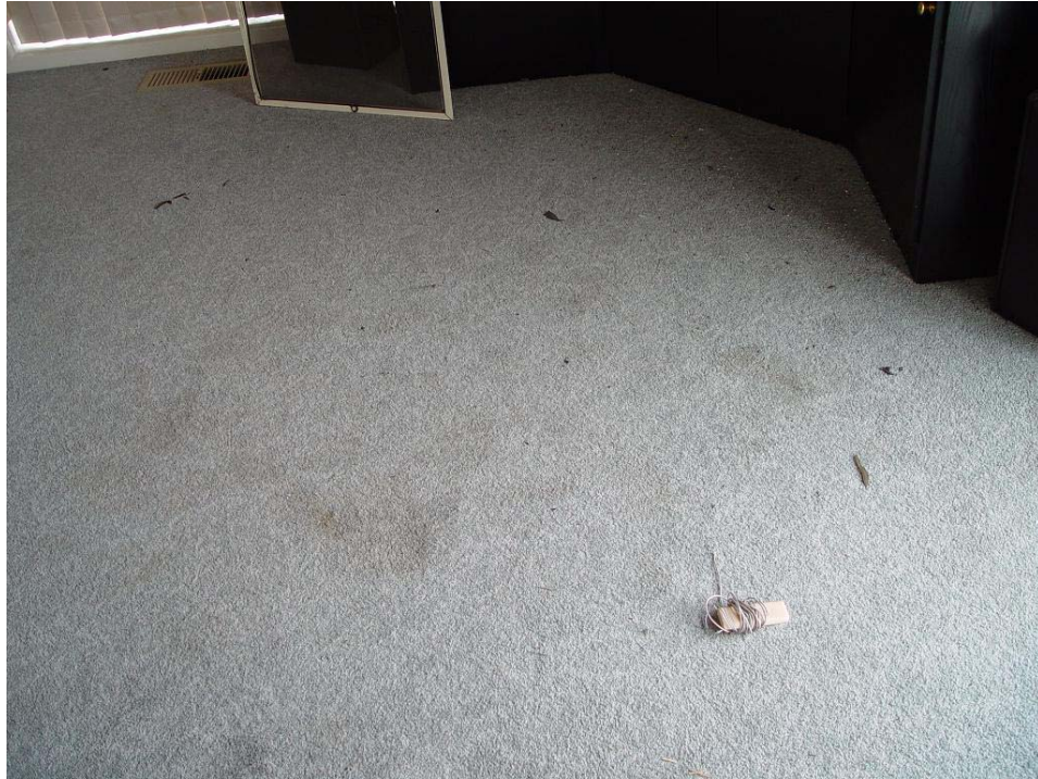
Figure 12. Ember attack on carpet (73 Somerset St)
