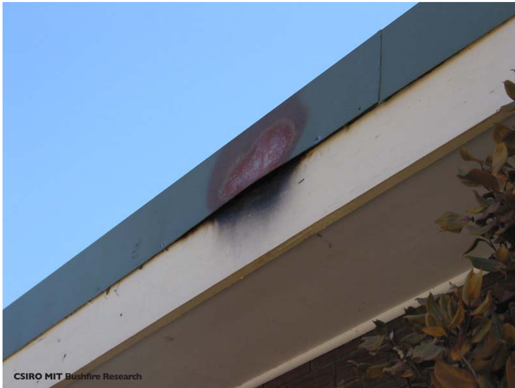
Figure 35. Ember attack on poor fitting capping
