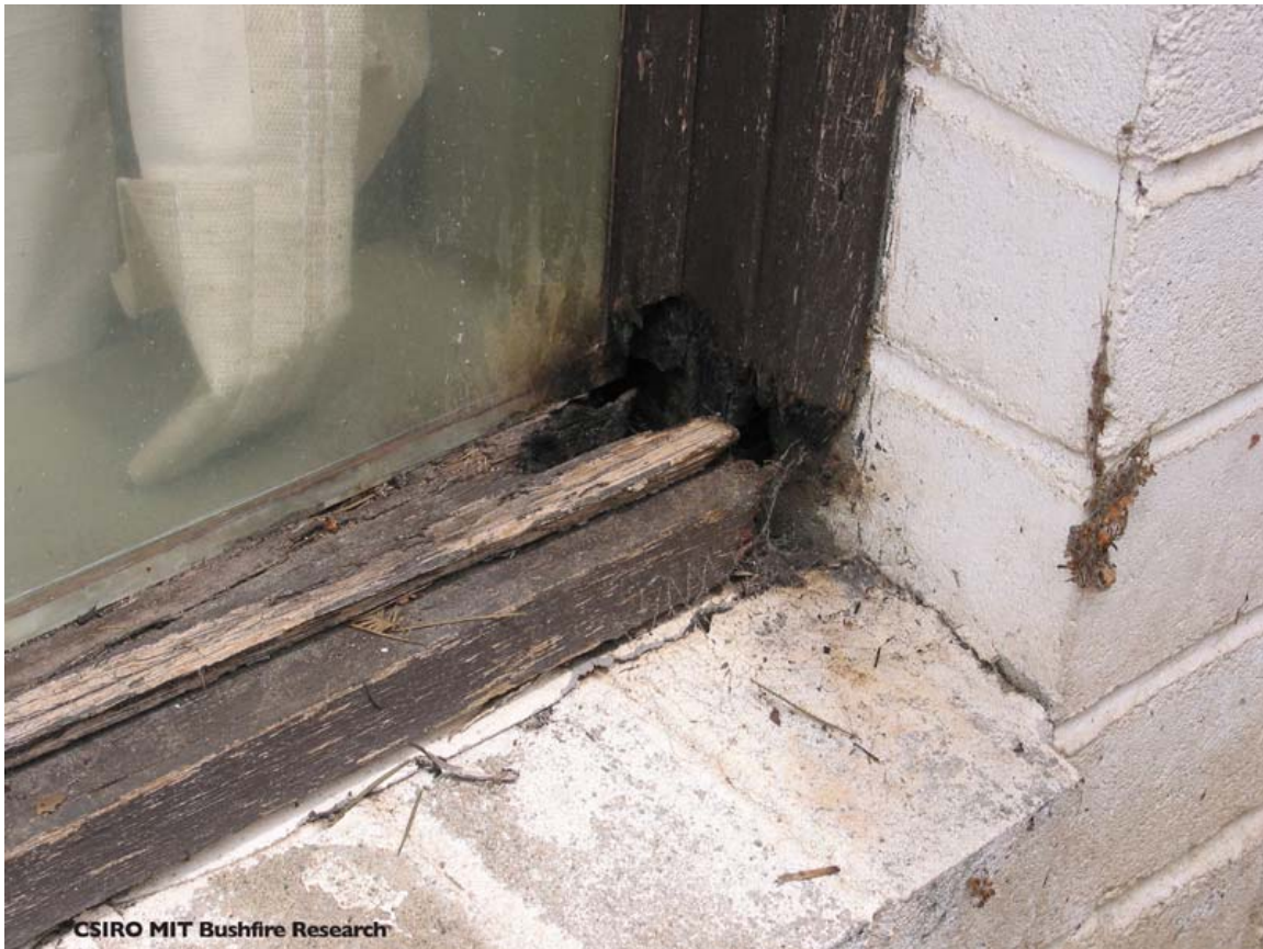
Figure 25. Ember attack at a re-entrant corner
