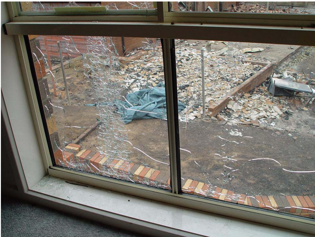
Figure 34. Damage to laminated glass
