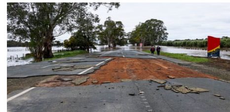
Flood damage to Midland Highway damage (Vic)
