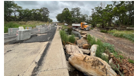
Flood damage to Comabella Causeway (NSW)
