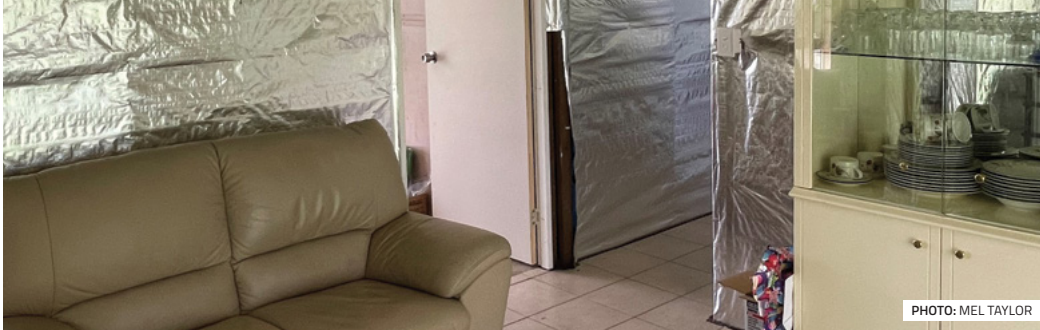
Rebuilding sections of a house after flooding.
