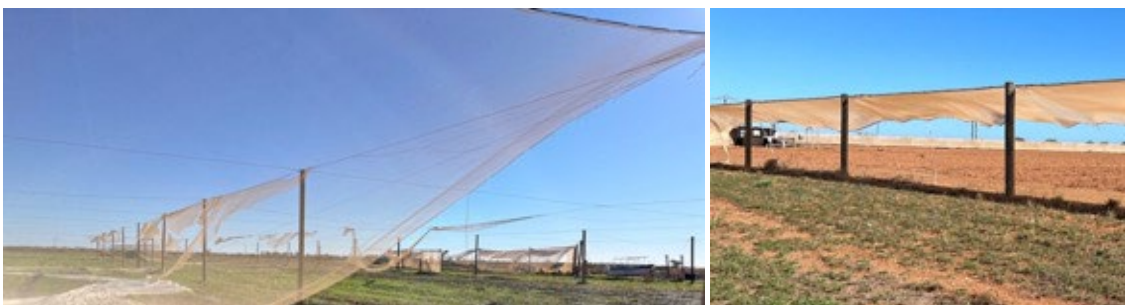
Damage to agricultural shade structures where they were not taken down prior to the event
