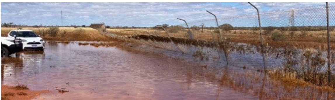
Storm tide mark on fence and damage in a carpark at Learmonth airport
